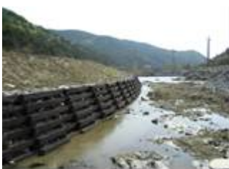
Construction d'éléments PE
