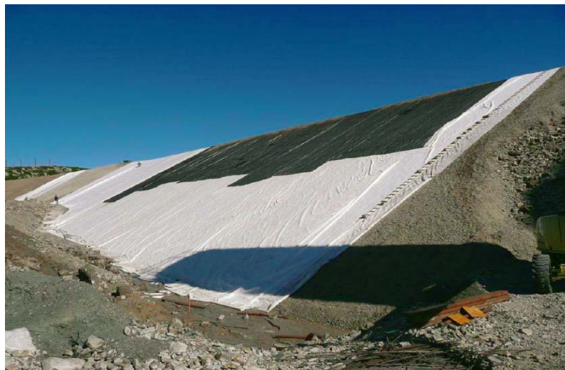
Figure 13. Installation du DEG
