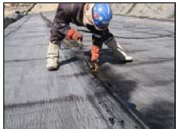
Figure 14. Finition du joint
