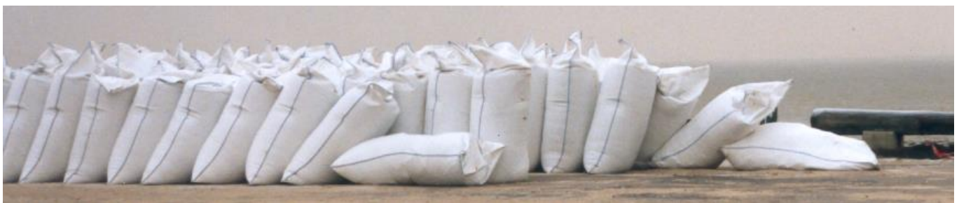
Figure 7. Conteneurs géotextiles (CGC).
